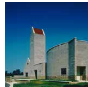
Unity of Dayton Church Ohio Masonry Council Award Huber Heights - Ohio 1987 Terry Welker FAIA, Architect of Record Co-designer: Michael Lebouf FAIA
