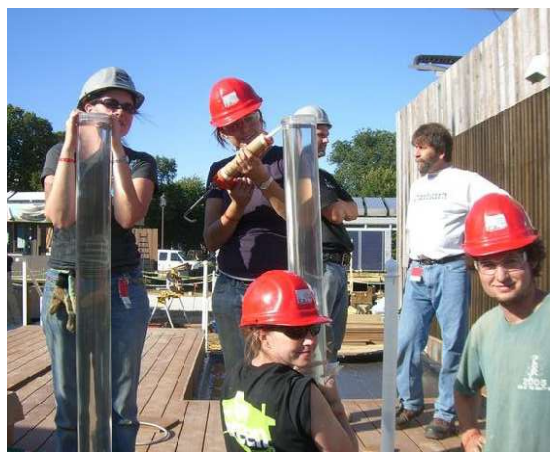
Clockwise from top: The Solar Decathlon Village on the National Mall, Washington DC. Filling the water tubes for the trombe wall. Shutters and sunshades help control heat gain while permitting air flow.
